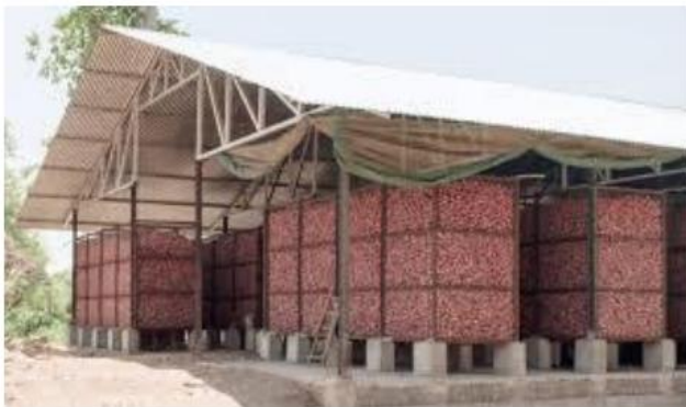
Fig:2 Traditional Onion Storage Structure Using Naturally Ventilated Storage Shed
