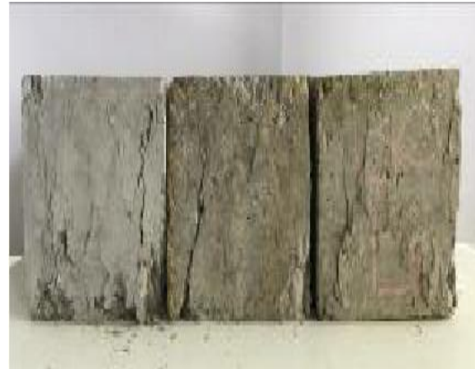
Image 3: Failure crack pattern of concrete cubes
